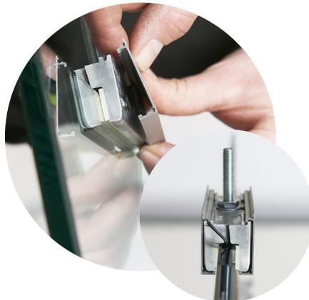
8 Fit the cover plates by hooking them on the top and pressing down until they click into the place against the glass.
