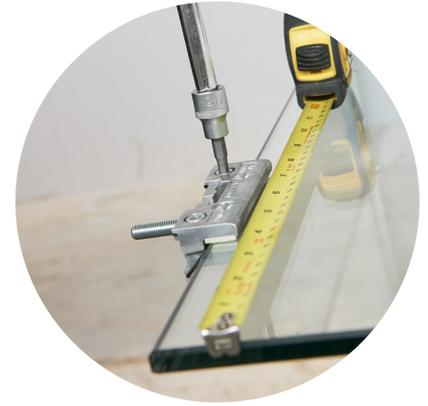
6 Fit the clamps 150mm from the edge of the leaf to the centre of the clamp.
